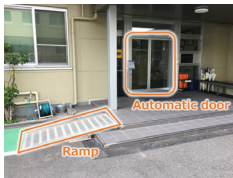
Office entrance and exit
