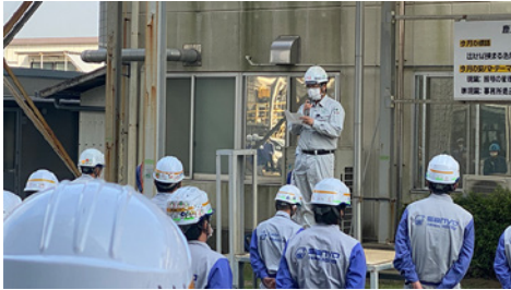
Kashima Factory: Safety talk by subcontractors
