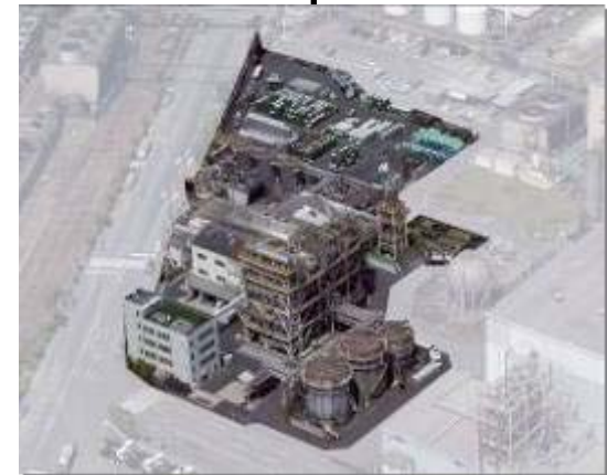
San Chemical Co., Ltd. Kawasaki Factory (Kawasaki, Kanagawa) Area: approx. 11,000 m 2
