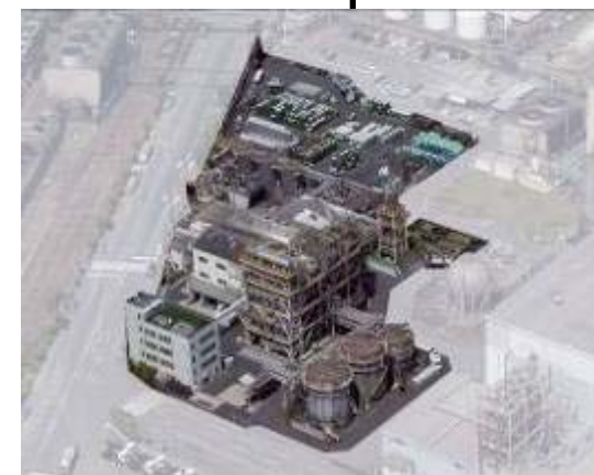
San Chemical Co., Ltd. Kawasaki Factory (Kawasaki, Kanagawa) Area: approx. 11,000 m 2
