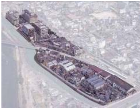
Kyoto Factory, Head Office and Research Laboratory (Higashiyama-ku, Kyoto, Approx. 26,000 m 2 )
