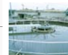
For wastewater treatment
